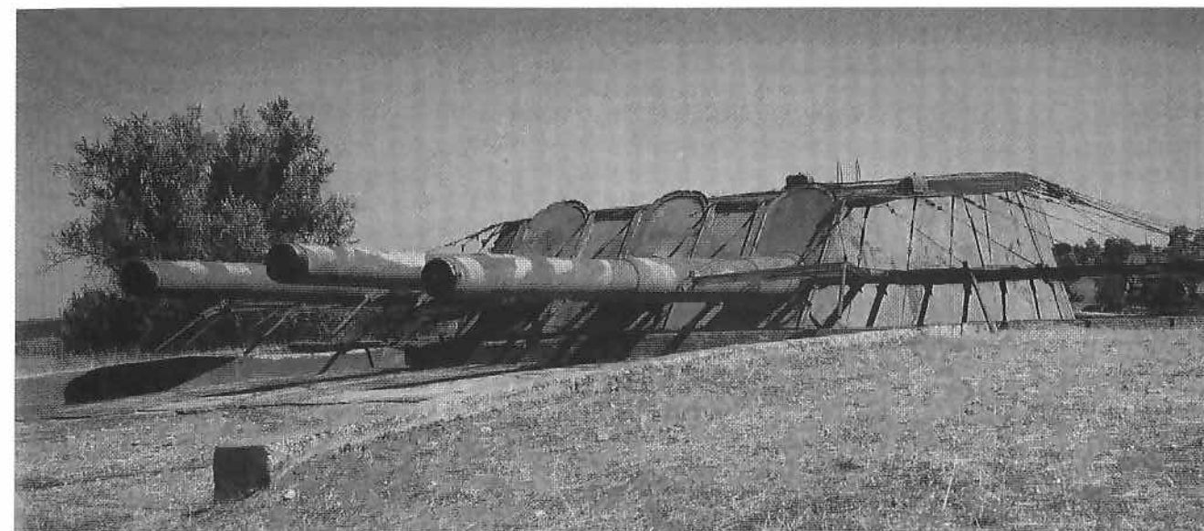
The eastern turret today, a nice comparison showing the main difference between the 'old' and the 'new' battery: although the type of gun — 305mm/52 M1910-1914 — is still the same,
