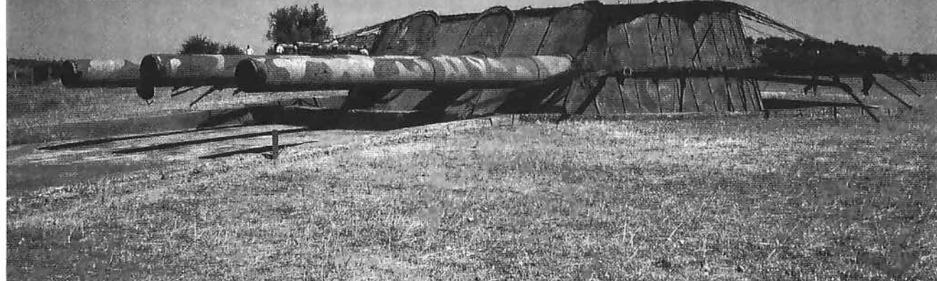
One of the strongest fortifications defending the Soviet naval base of Sevastopol on the Crimea during the seven-month German siege of the city was Battery No. 30, known to the Germans as Maxim Gorkii I. Its powerful 305mm guns battered by super-heavy artillery and aerial bombardment, it was finally captured in a frontal assault in June 1942. Rebuilt and modernised after the war, the battery is still an active military installation of the Russian army today.
