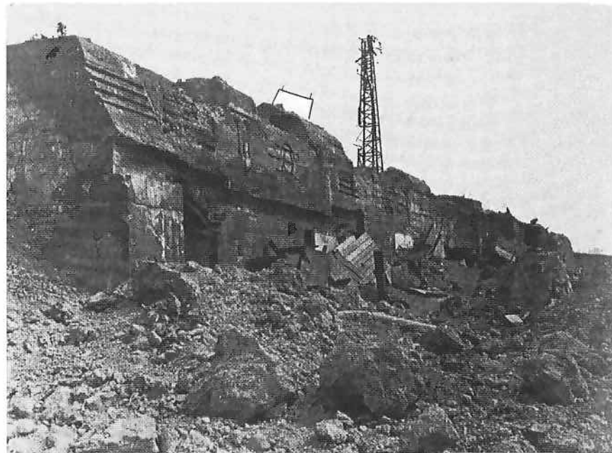
Rocks and debris obstruct the entrances to the battery block. With all guns silenced, and their escape route via the tunnel blocked by the Germans, the 230-strong Russian garrison was bottled up inside the fortification. Those wanting to surrender were kept from doing so at gunpoint by political commissars, and it was three days before they came out. By then, half the garrison was dead. Picture by PK photographer Horter. (NIOD)
