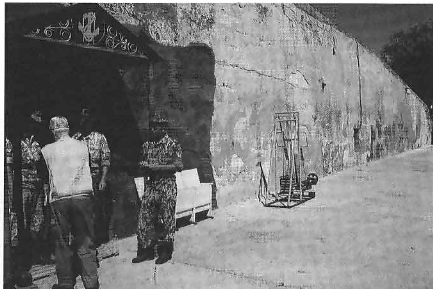
The entrance to the gun casemate as it is today. Compare with the picture at the top of page 50. The exterior facade looks different because an extra layer of concrete was added in 1950-52 to increase strength. All present-day photos by Svein Wiiger Olsen.
