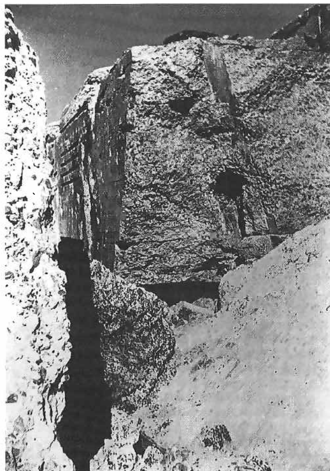
The gun casemate of Maxim Gorkii I was deeply entrenched in the rock and its concrete walls were several metres thick. Another picture by PK photographer Rauchvetter. (NIOD)
